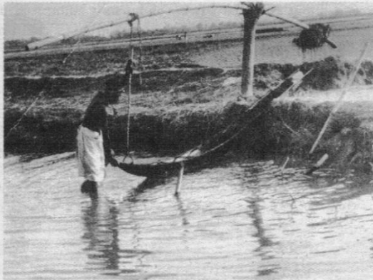
Fig. 3.2. Don used to lift water from a shallow stream.
