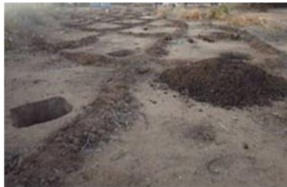
Fig. 32.1. Negarims under construction. (Source: Critchley, 1992)
