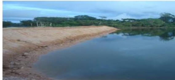
Fig. 4.10. View of a Detention dam.
