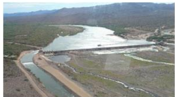
Fig. 4.9. View of a Diversion dam.
