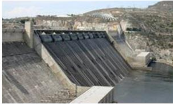
Fig. 4.3. Photograph of a Solid masonry gravity dam.
