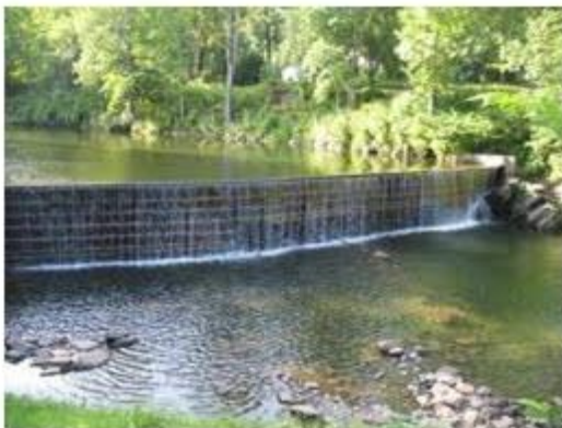
Fig. 4.6. View of a timber dam.
